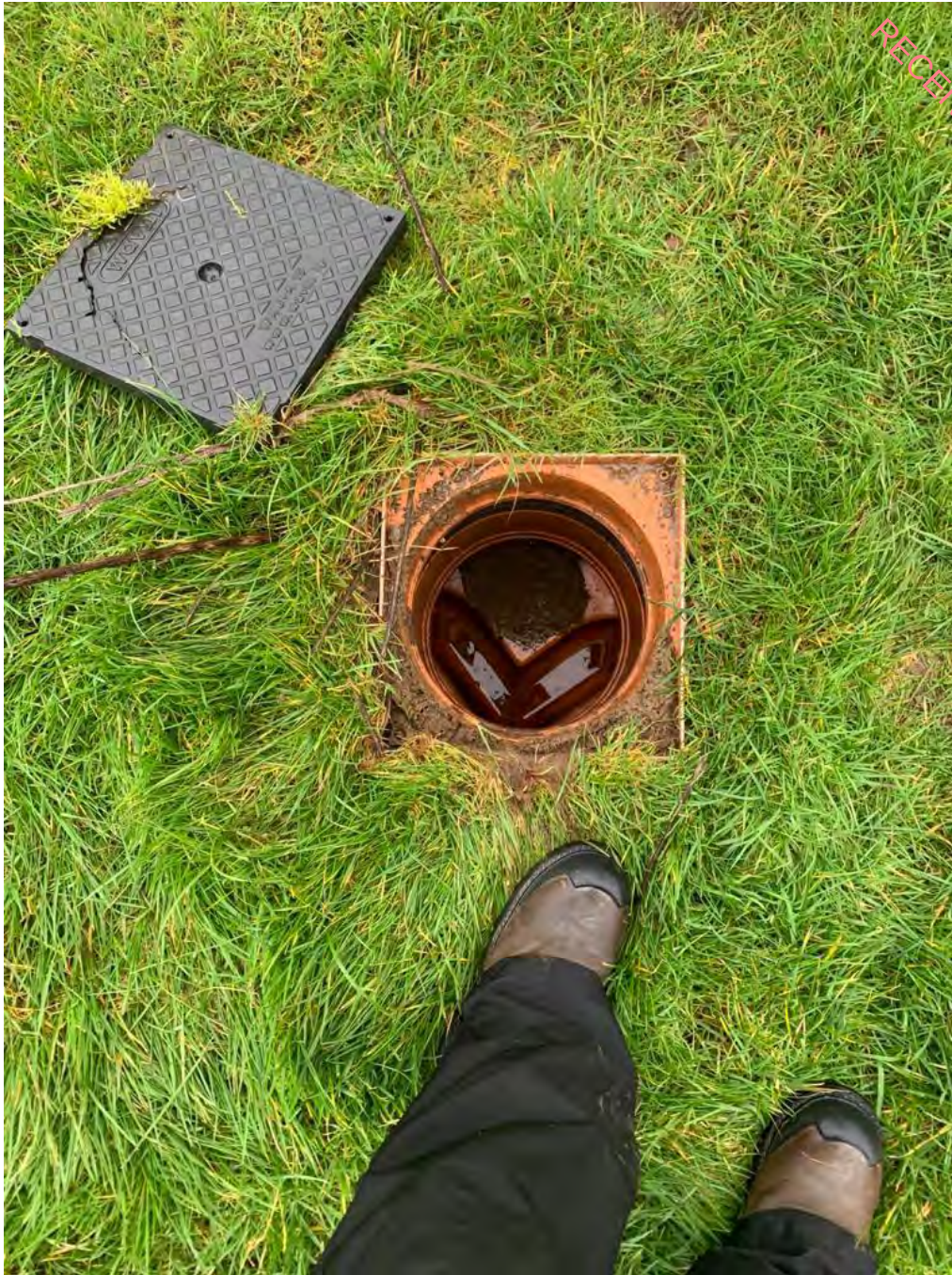
Photo 7 Splitter box view = clear treated wastewater.
