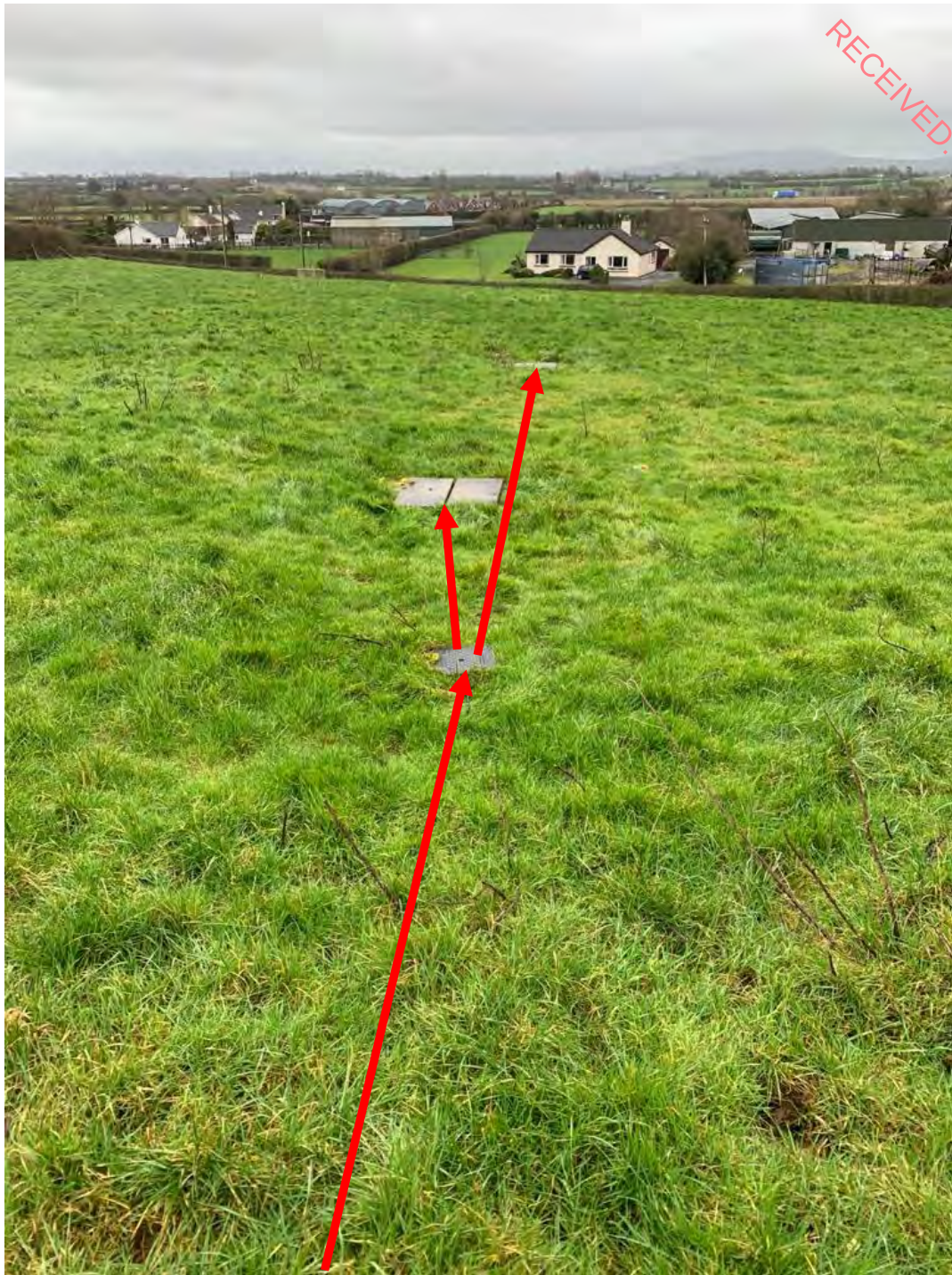
Photo 6 Line of 100mm PVC plain walled sewer pipe conveying secondary treated WW from the Puraflo modules to the splitter box that feeds both distribution boxes, which in turn feed four percolation pipes and associated trenches.
