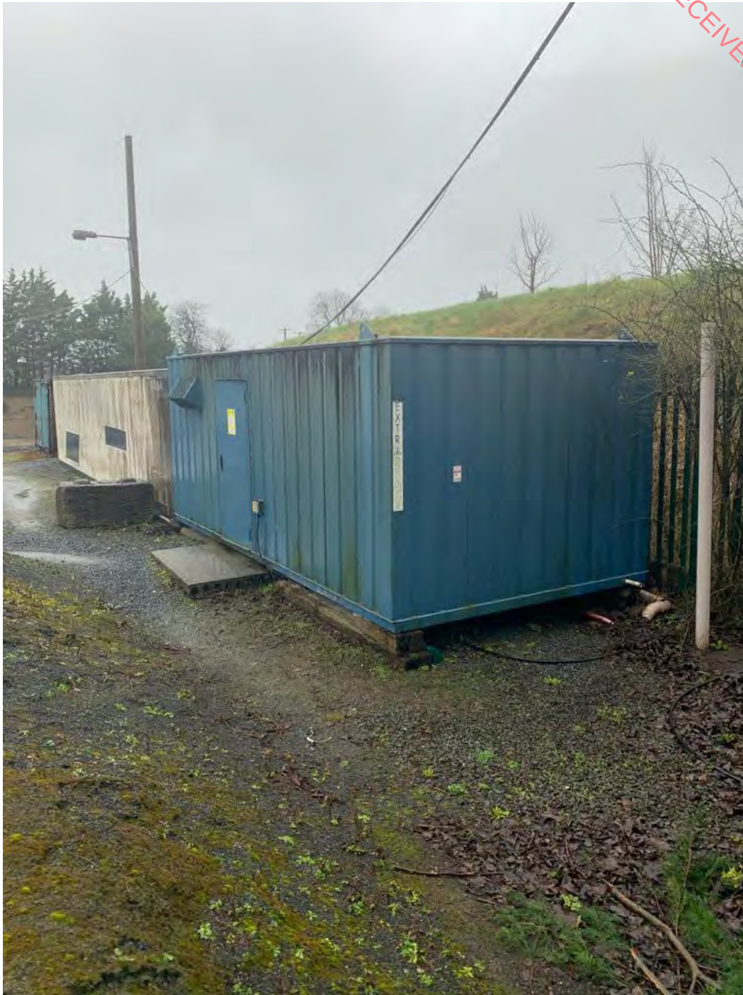
Photo 5 Quarry Floor Staff Toilet & Septic Tank Vent adjacent (at the base of the hill that homes the PuraFlo modules).
