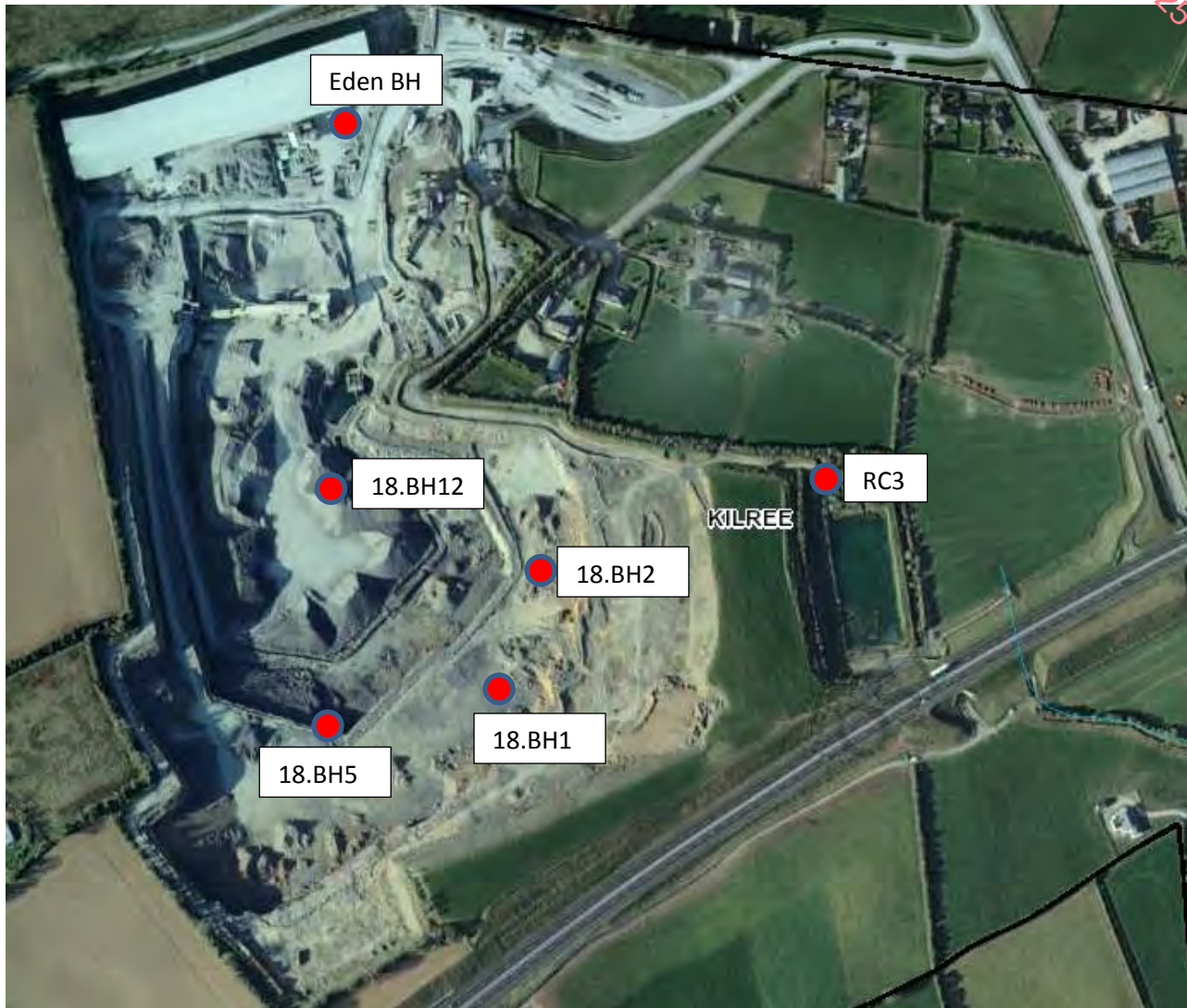
Figure 1 On-site Water level datalogger locations.
