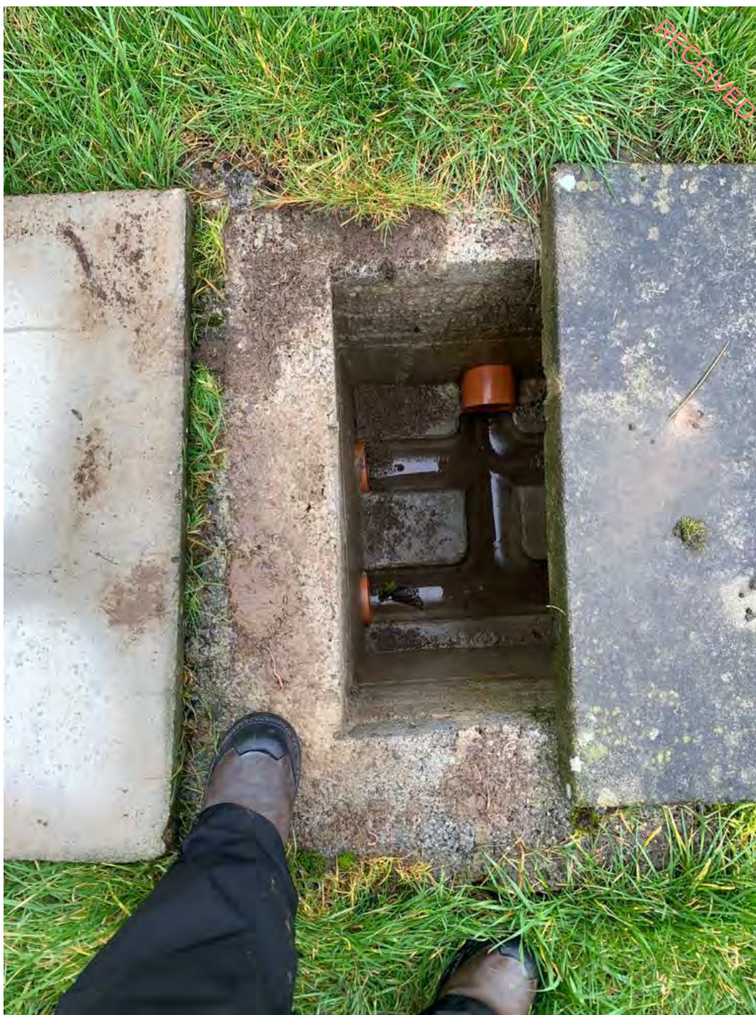
Photo 8 One of 2 no. distribution boxes: clear treated wastewater.
